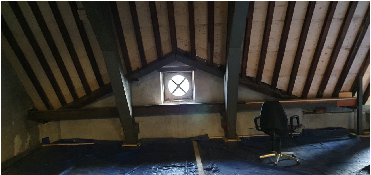
Wooden water collector in the attic of the Dedel house.
