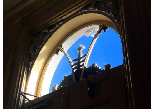
Hallway door window [image 4]
