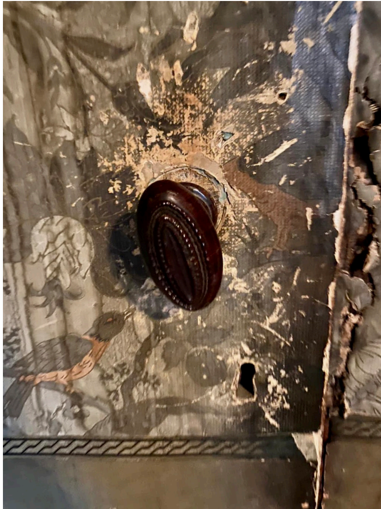
5. Fragile condition of the doorknobs, House Dedel.
